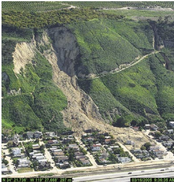
On Jan. 10, 2005, a landslide struck the community of La Conchita in Ventura County, destroying or seriously damaging 36 houses and killing 10 people.
