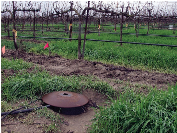
▲ A sump pump was used to monitor runoff from storm events, as well as collect water samples for sediment and nutrient analysis.
