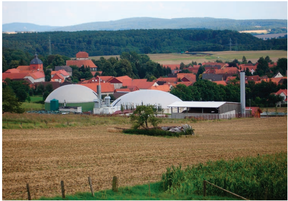
Covered lagoons and methane digesters are an option for reducing greenhouse-gas emissions from dairy waste. In Germany, the village of Juehnde built a digester for livestock waste and other biomass. The methane is combusted to produce electric power and heat for homes in the village, which is the first in the world to go “off the grid” through the use of its own waste.
