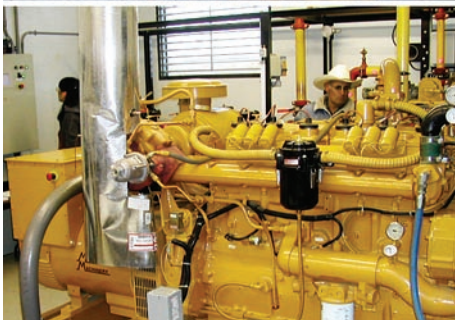
Top, manure from dairy cattle is used as a feedstock for anaerobic digestion to produce biogas (primarily methane and carbon dioxide), which, above, generates electricity at the Castelanelli Dairy in Lodi.
