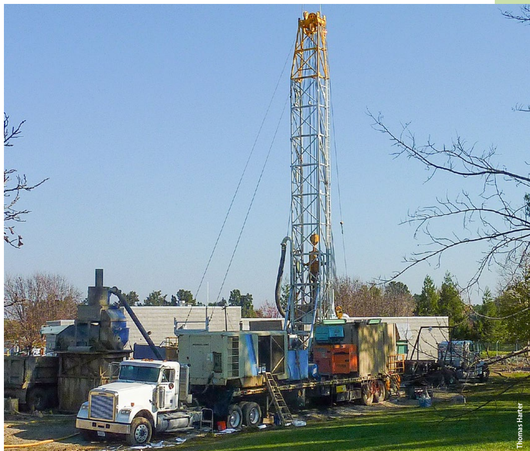
Water well drilling rig on the UC Davis campus.
