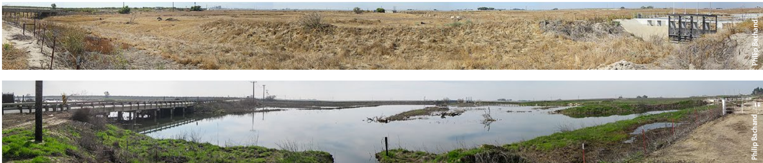
Panoramic picture of the James Bypass from the Terranova Ranch in October 2010 (top) and early February 2011 (below) from the Highway 145 overpass to the James Weir. Flood flows occur approximately on a 2-year interval, but the James Bypass can be dry for years at a time or flooded for several months consecutively.
