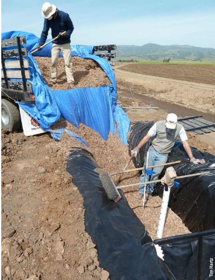
Denitrification bioreactor being filled with wood chips.
