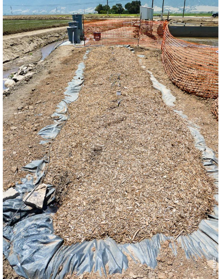
Completed denitrification bioreactor.
