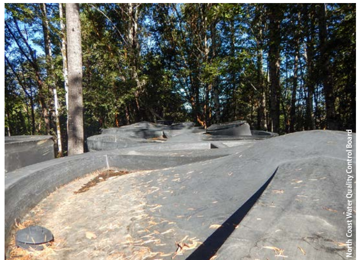
Rainwater catchment. Storage tanks with filtered tops are one of many means for collecting rainwater.
