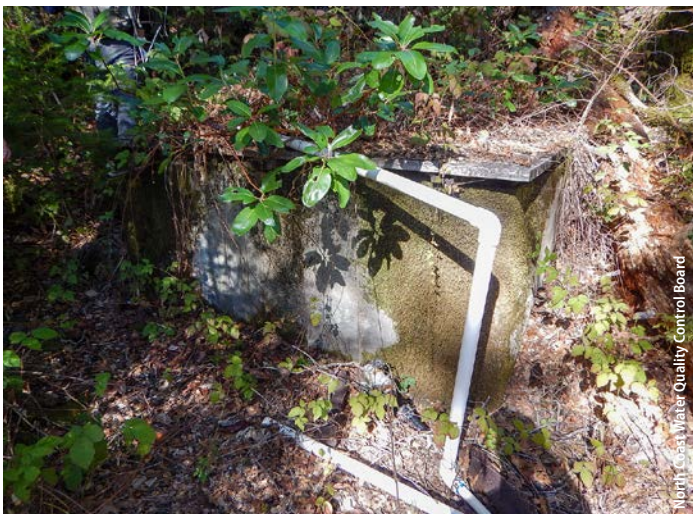
Spring diversion. Spring box installed to consolidate flow, which is then directed through PVC piping.
