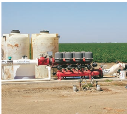
Left, A set of filters prevents irrigation water from clogging the drip lines. Right, Pressure-regulating valves allow growers to control the pressure of the irrigation water flowing into the drip line.
