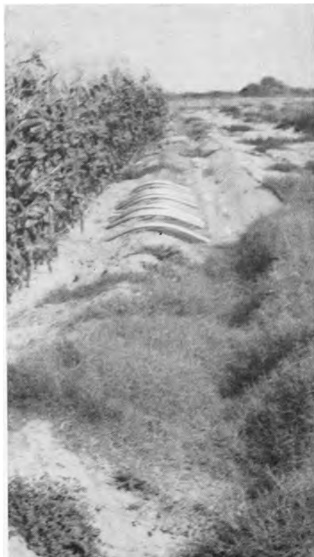
Use of siphons in ditch with vegetation controlled by lining.
