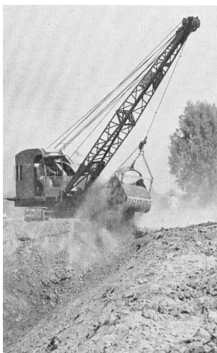
Dragline excavating a drainage ditch.
