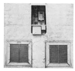
Modified form of "Champion Fly-insect Electrocutor" installed in the vent openings.
