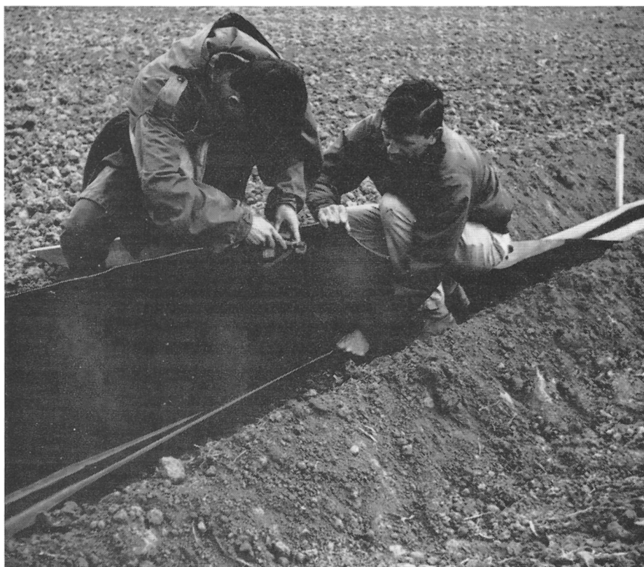
Plastic film being installed in 1961 field trials for water control in rice irrigation.
