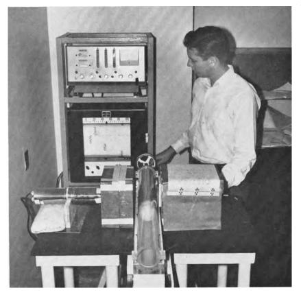
The ability of soil to transmit water affects the rate, frequency and method of irrigation—and can often limit cropping possibilities in non-irrigated areas. Knowledge can be obtained on water movement through soil by measuring changes occurring after different peiods of time. The gamma ray apparatus leasures soil moisture on the basis that ewer gamma rays will pass through a ret soil than a dry soil.
