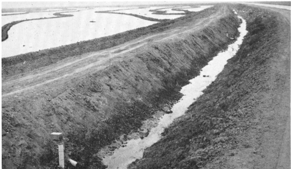
The leaching operation on the land following installation of the tile drains. Rice was planted in the spring of 1963, following leaching.
