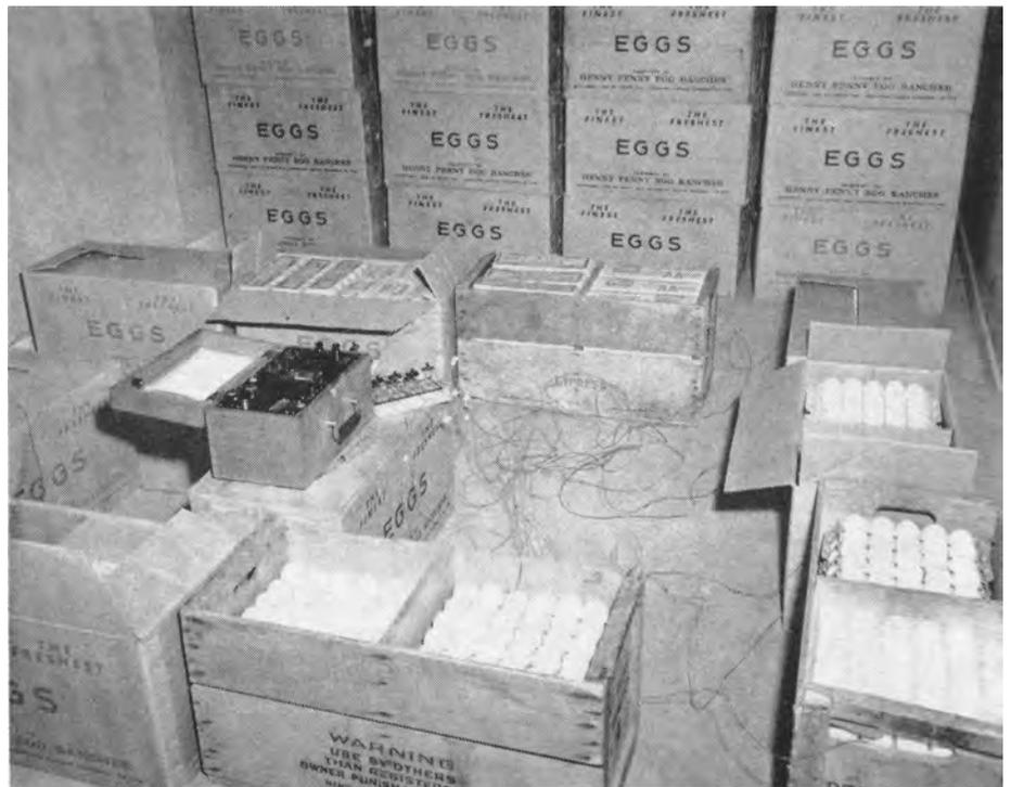
“openness” of the container and (2) air circulation. In a conventional cold room without a forced air cooling system, the eggs must be placed in open containers such as stacked filler flats if the cooling time (to 60° F) is to fall within the recommended 8 to 10 hour limit. Placement of eggs in tight containers such as the closed fiber cases will result in excessively long cooling periods even where the cases are not stacked.
