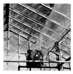
Poly-tube ventilator in greenhouse.
