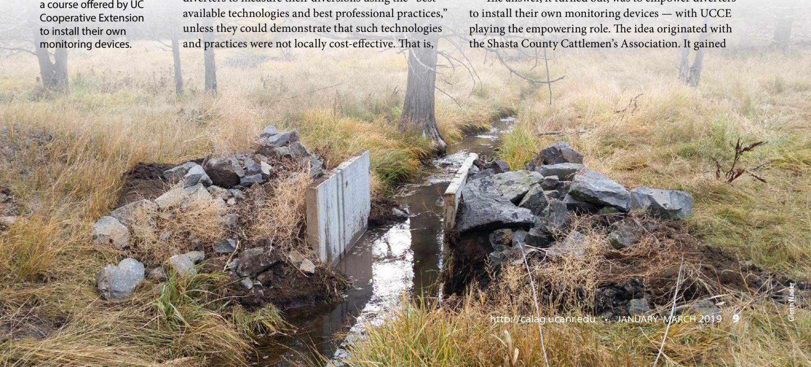
A weir at the UC ANR Sierra Foothill Research and Extension Center in Yuba County. Once installation of a monitoring device for a weir is complete, water diverters need only read a staff gauge that shows the height of the water spilling over the weir's crest — and do a bit of math.
