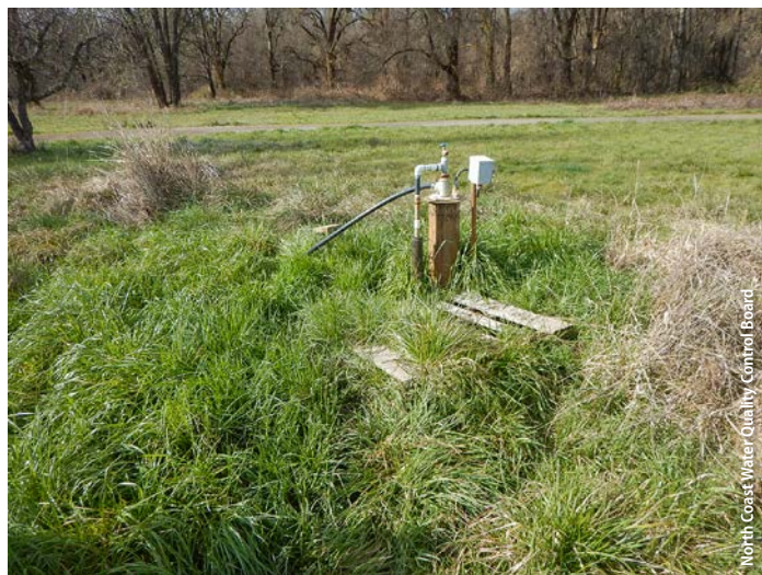
Subsurface water well. Well casing with associated power box and piping, used to convey water to storage or used for direct application.
