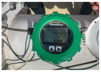
Accurate water monitoring is a first-order concern to ensure functioning groundwater markets. Meters, in place on Fox Canyon groundwater wells since the 1980s, track water use, left. To prevent cheating and ensure accurate data collection, Fox Canyon growers opted for universal telemetric sensors that attach to meters and stream pumping data real-time, funded by a grant from the Natural Resources Conservation Service, right.
