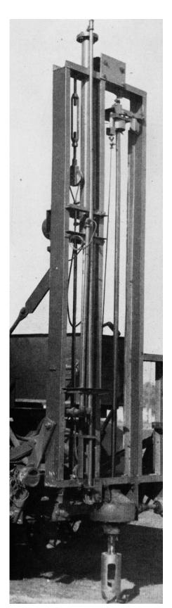
Power-operated Soil Sampler
