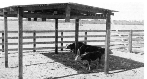
Cattle standing under shade covered with 1" x 10" boards spaced 1" apart. Air temperature 103° F and ground temperature in shadow 104° F. In unshaded strips between board shadows, ground temperature was 148° F. High ground temperature may be reason for cattle not lying down.
