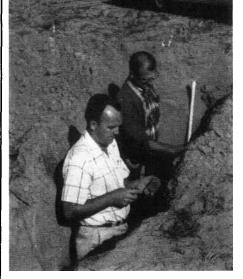
Observations of soil compaction and water penetration problems in orchard photo above were made possible by backhoe trenching.
