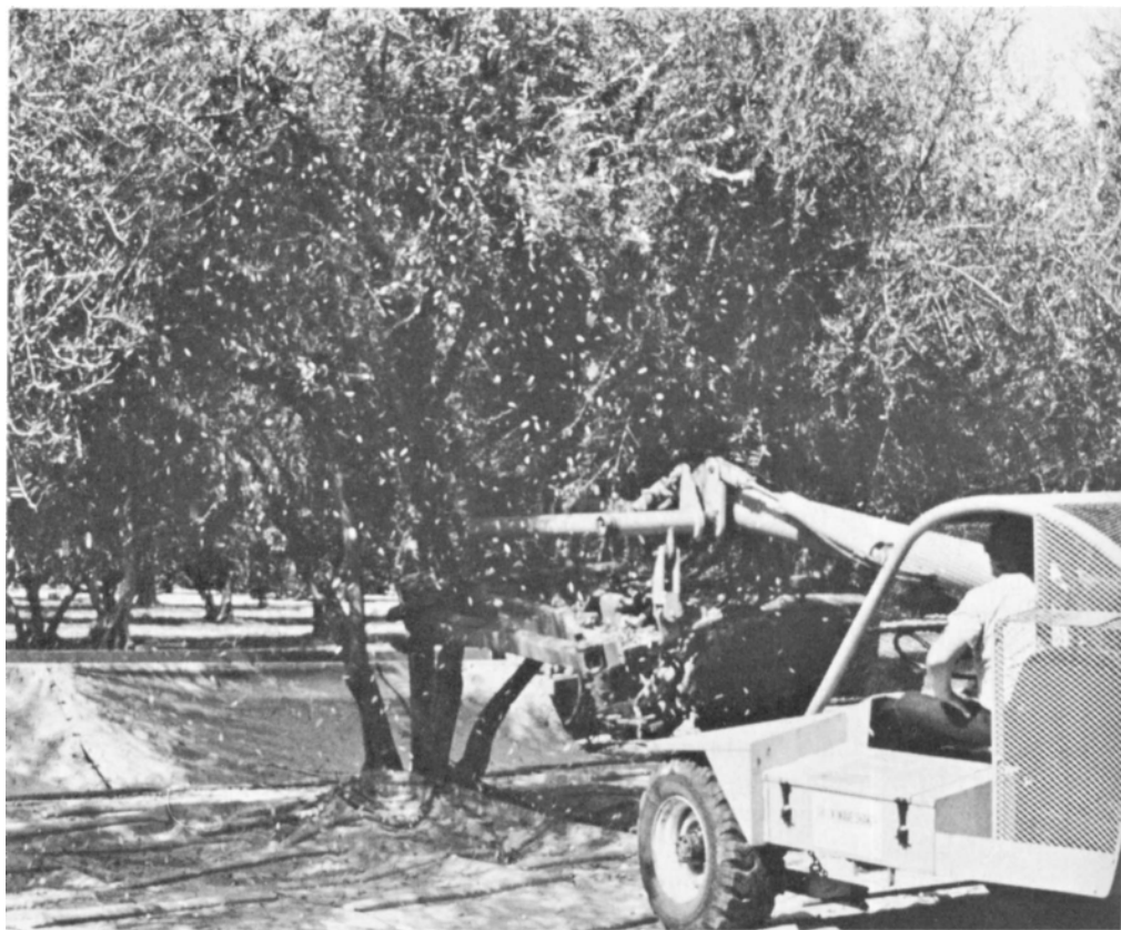
Photo 2. Tree shaking equipment in action on a well-prepared tree. Fruit is being caught on a mechanized, roll-out, canvas catching frame.
