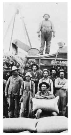
This threshing crew poses in front of its thresher built around 1900 by the Advance Thresher Company of Battle Creek, Michigan. Operated by PTO (power take-off) belt, the separator, by means of a series of shaking screens, separated the grain (in bags, foreground) from the straw.
