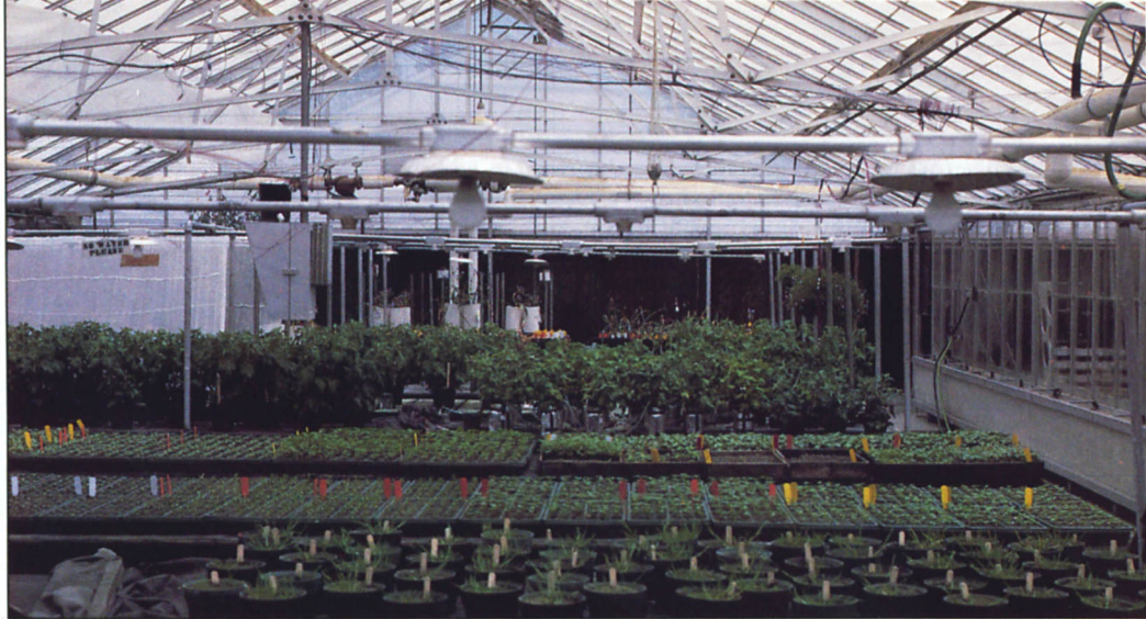
Bench-top heating required less energy than the conventional perimeter heating system in this commercial greenhouse, but provided less uniform temperatures in the plant canopy.
