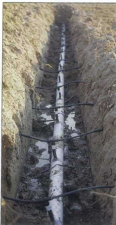
Four-inch sub-mainline is shown in a trench which runs across the furrows. Lines of drip tubing which have been shanked under the center of each 40-inch cotton bed are connected to the sub-mains before burying the line.
