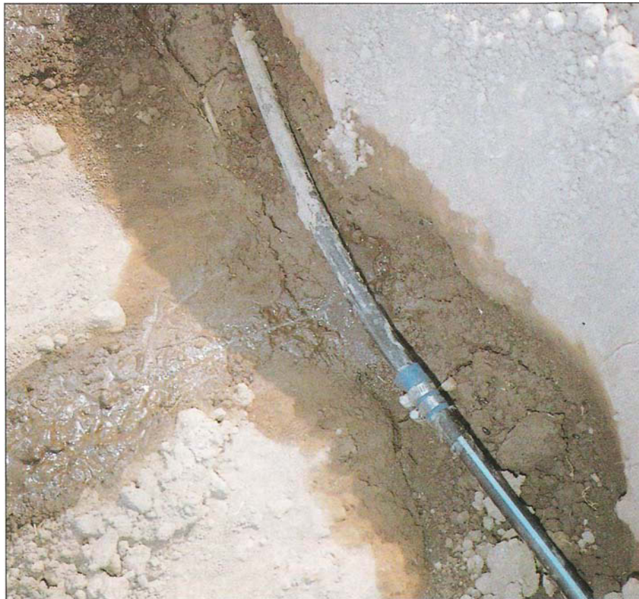
Soil has been excavated to reveal drip tape installed and operating.
