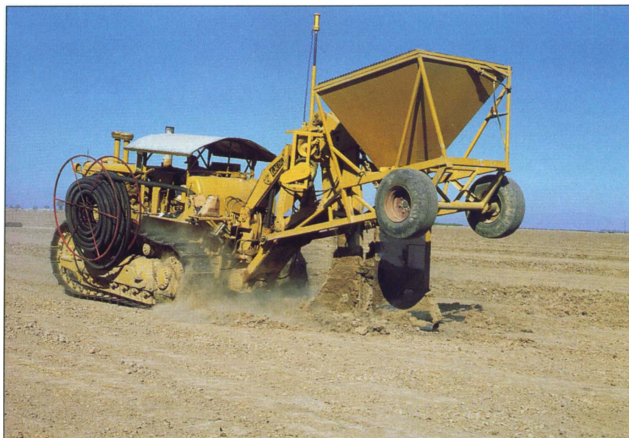
Replacement of old clay and bituminous fiber drains with new plastic drains only increased drain flow rates, rather than improved drainage of the field.
