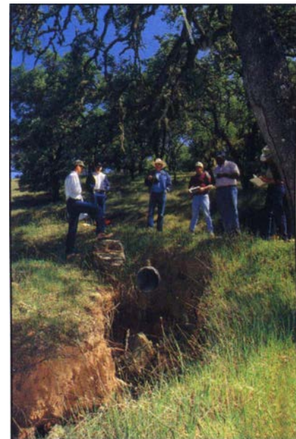
Culvert water concentrates intermittent high periods of runoff creating a "headcut." Left unchecked, headcuts can carve deep into a hillside, damaging vegetation, increasing erosion and, in severe cases, lowering the water table.
