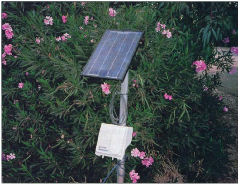
In some soil types, the Enviroscan readings were inaccurate.
