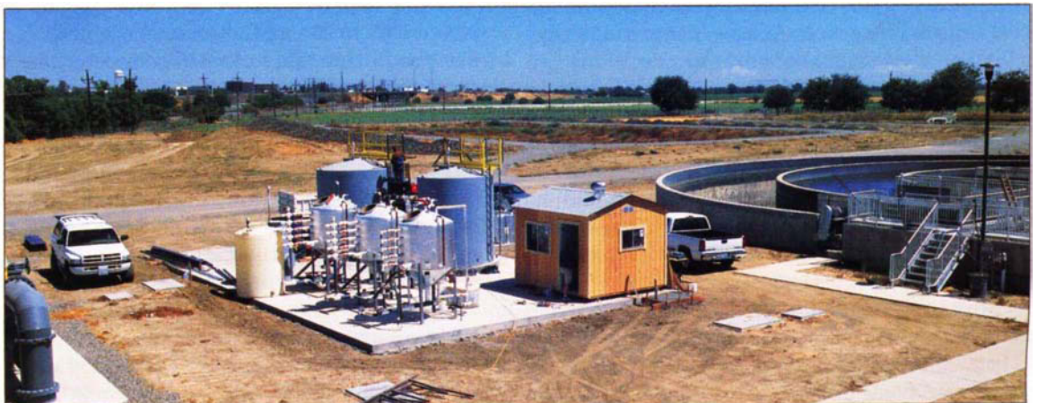
At UC Davis, a pilot plant is under construction of the APS-Digester, which converts animal manure and plant waste into biogas under anaerobic conditions. The first commercial application will be at a Florida racetrack, but it has broad applications for dairy, swine, poultry and other animal operations.
