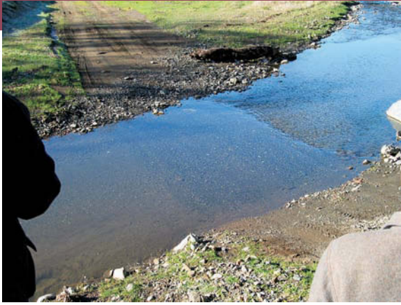
Road crossings at streams are an important source of potential sediment on North Coast rangelands.
