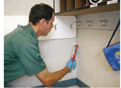
The UC Statewide Integrated Pest Management Program (UC IPM) is working with the California Department of Pesticide Regulation to train school-based IPM coordinators in less-toxic pest control methods. Top to bottom , a school IPM coordinator applies boric acid powder to cabinet voids in the school kitchen, monitors for pests, places sticky traps for roaches and caulks to exclude ants.
