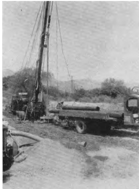
Drilling an experimental drainage well.
