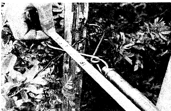
Figure 19. — Measuring from the fencepost to the end of the tension spring.
