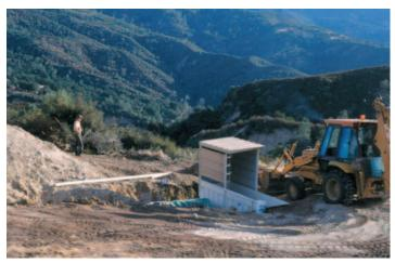
Figure 30. Deer guzzler under construction, San Benito County, California. The collection apron will be installed over the underground storage tanks (left of the access ramp) (Photo by Phil Pridmore/CDFG).
