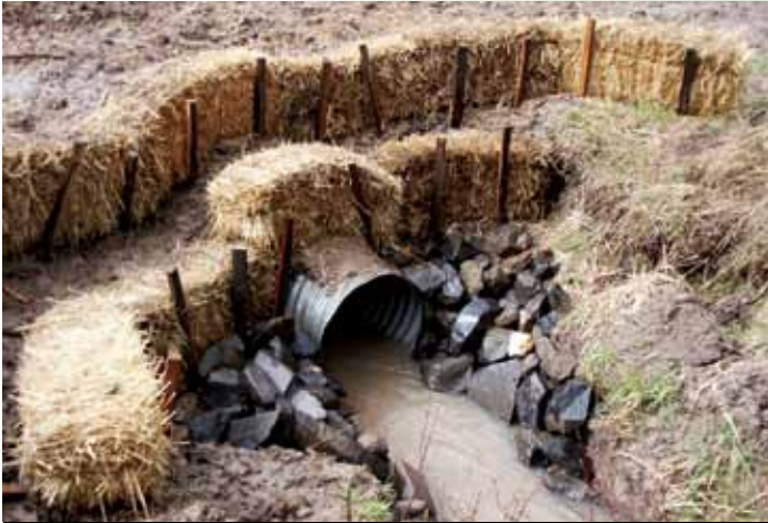
Properly installed and protected culvert.
