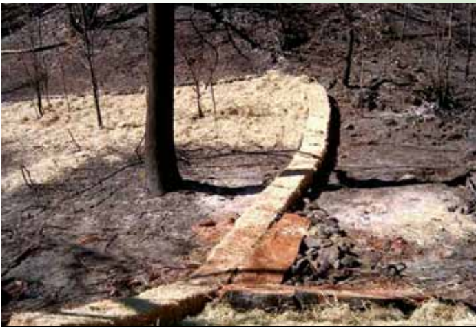
Straw bale check dam.
