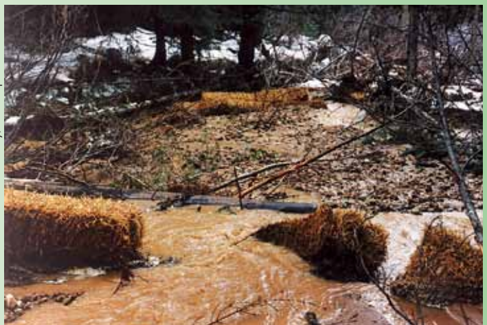
Failed straw bale check dam.
