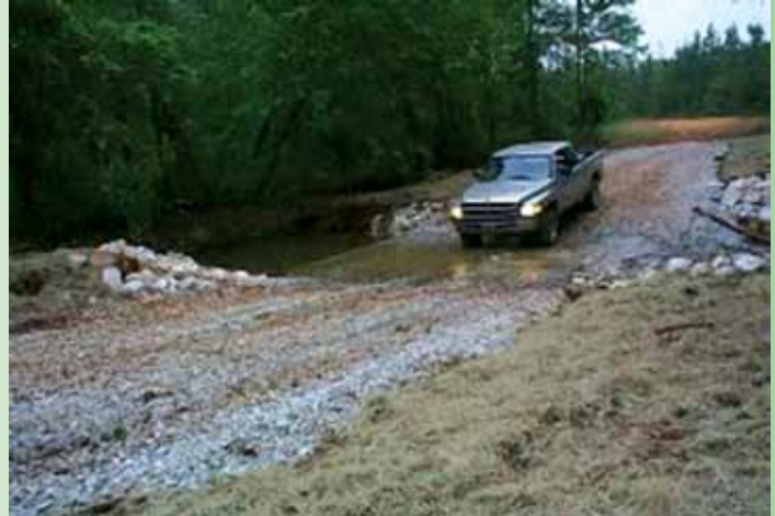
Armored stream crossing.
