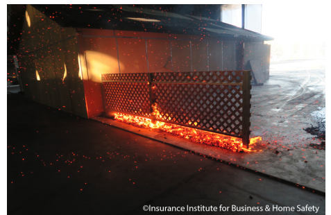
Flame spread to the building occurred more easily when combustible debris was present at the base of the fence, as shown here.
