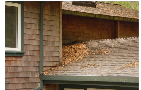
Replacing siding "locally," in areas where it meets the roof on a complex roof design, such as that shown here, would be more affordable than "global" replacement. Source: Stephen L. Quarles
