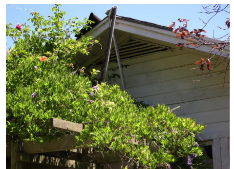
Vegetation growing over a trellis structure. If ignited, flames would impinge on the side of the house, including the nearby gable end vent. Source: Stephen L. Quarles
