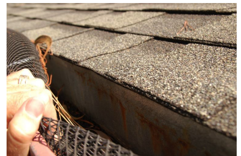
Gutter with integrated drip edge. Source: firecenter.berkeley.edu/bwmg/gutters.html
