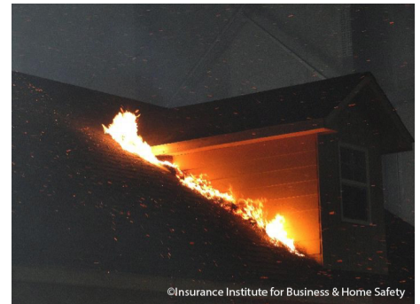
Wind-blown embers ignited debris on a roof next to dormer.
