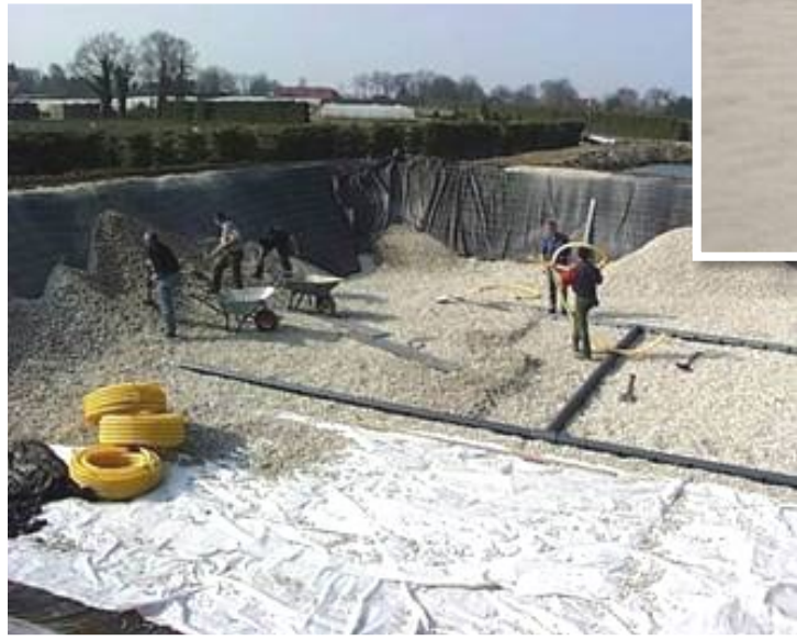
Underdrain system (lowest level)
