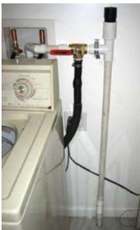
Laundry to landscape system, showing diverter valve and vacuum break vent. Vent would have been best placed outside to prevent flooding though. Pipe shown goes through floor and out to mulch basin. Uses machine pump but be careful not to go too high.
