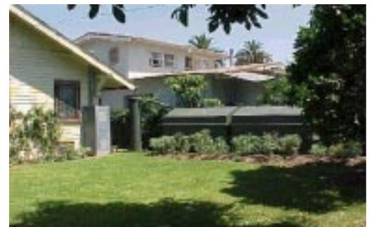
System for collecting and storing storm runoff from a residential roof.
