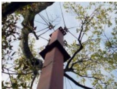
*Closeup view of tower and cable system installed to support specimen live oak.*
