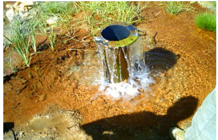
UNCONTROLLED LEAKAGE FROM ARTESIAN AQUIFER SYSTEM
