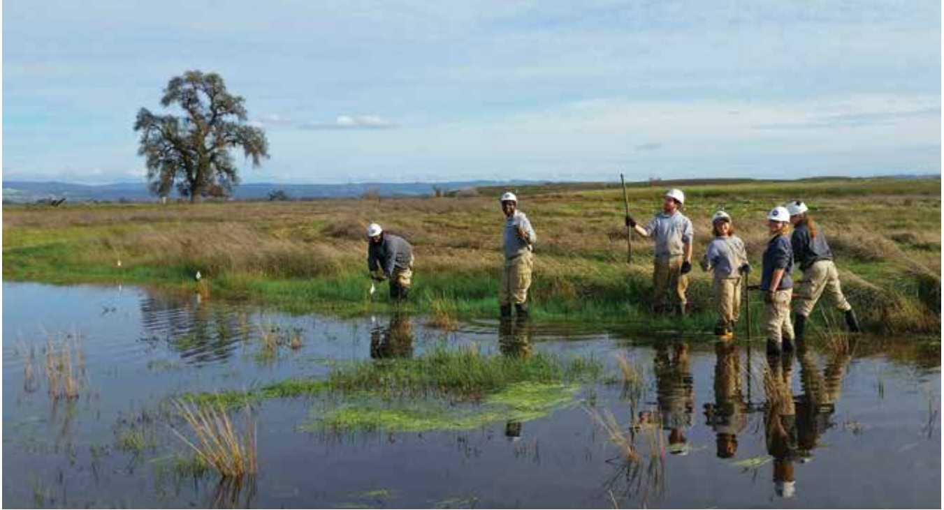
FIGURE 14. b) Work crew planting the stakes along a creek in Placer County.
