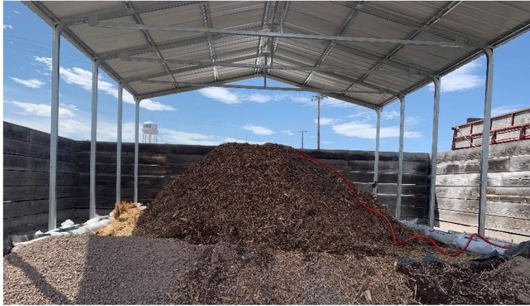
An existing 3-sided structure with cement at the base was retrofitted to accommodate the permitting regulations for the composting pile. A metal roofed carport structure was installed within the structure as a roof, required by the regional water quality board. Base rock material was placed on the floor and a pond liner was put on top of the rock to act as an impermeable layer. Then tube sand was used to secure the pond liner and created a basin to deter any runoff from the site.
