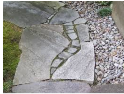
Figure 2. A stone pathway and rock mulch has been installed to create a non-combustible zone. (Photo by El Dorado County MGs)
