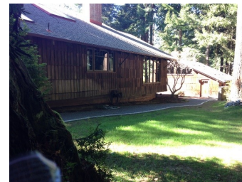
Figure 1. Vegetation has been separated from the house and its combustible siding by installation of an asphalt walkway.
