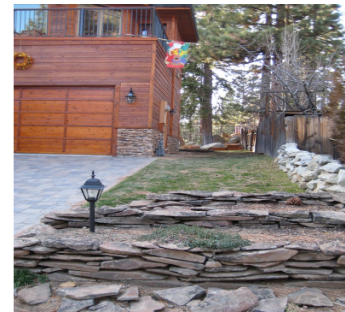
Figure 3. Rock mulch has been extended around the base of the house. Stone facing at the base of the house reduces the risk of having combustible wood siding.
