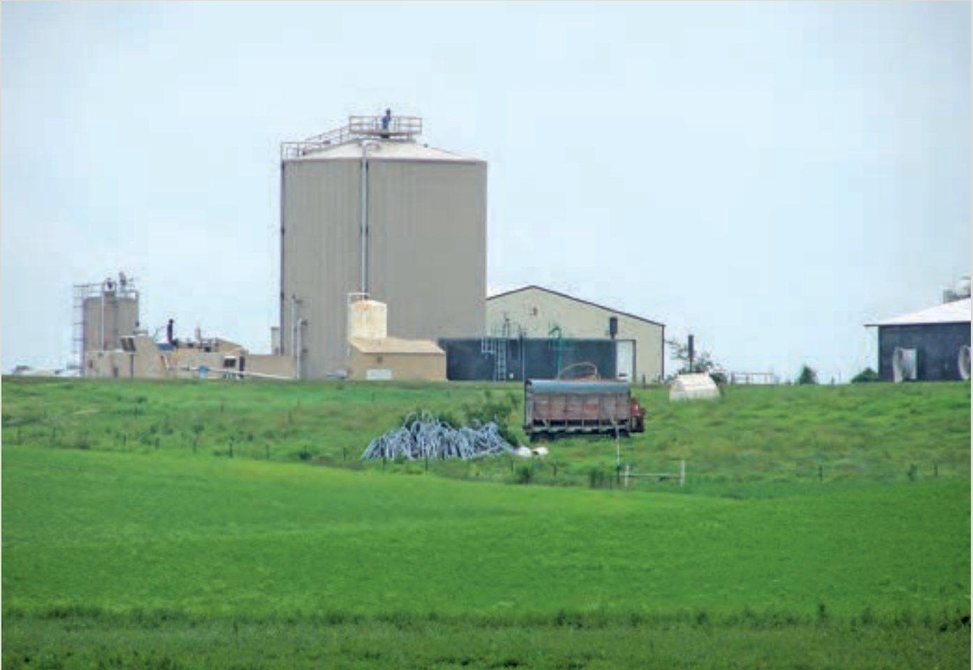
Anaerobic digester at Five Star Dairy.
