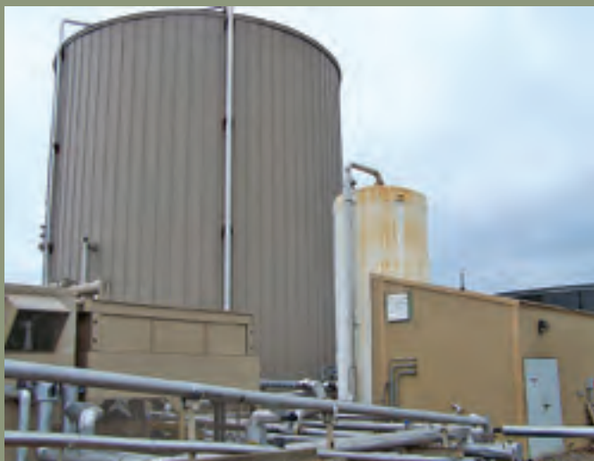
On farm anaerobic digester located at Five Star Dairy in Elk Mound, Wisconsin.
