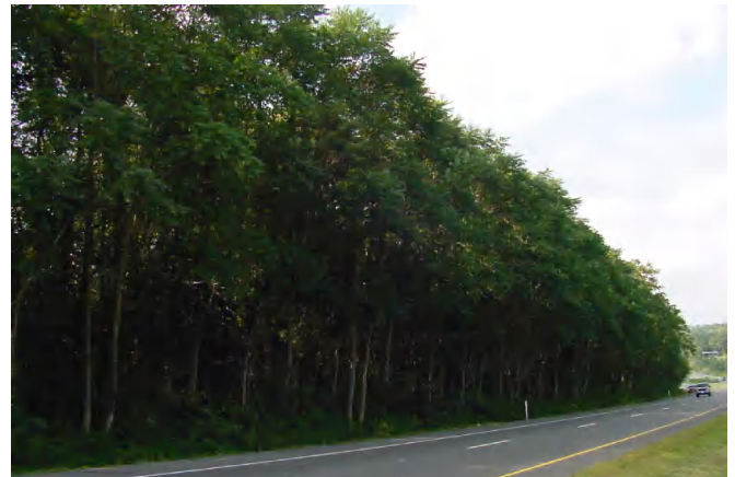
Figure 1. Due to its rapid growth, tree-of-heaven, or ailanthus , can quickly become established on the right-of-way. Unless aggressively managed, it will quickly grow tall enough to impede sight distance, become a collision target or tree-fall hazard.
