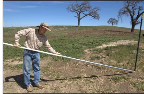
Insert the bottom end of the "Mr. Longarm" into the line post; it should insert 2 ft. inside the post, and the band of "Gorilla" tape should be fully inserted inside the line post with a fairly close fit. If the fit is too loose, add more "Gorilla" tape; if too tight, remove some of the tape.
